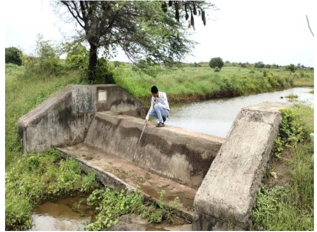
Survey of Water Harvesting Structures
